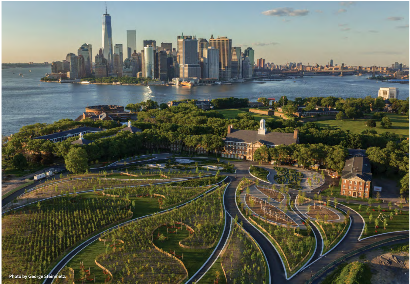
Aerial view of Governors Island, with a mix of young and mature trees, looking toward lower Manhattan.
