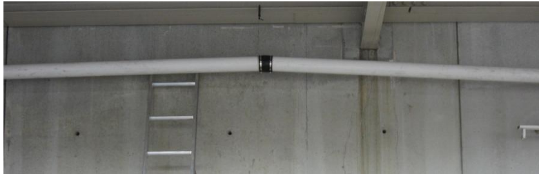
DO NOT pitch pipes upward.
