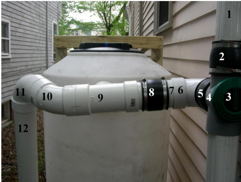
This design uses the same tank opening for both the inflow and overflow.
