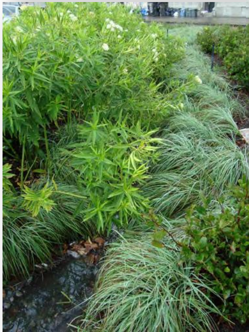
Figure 2. Greenstreet at Church Avenue inlet in Brooklyn, NY, constructed in spring, 2009. Curb cuts direct stormwater runoff into the bioretention area. Photo credit: Nandan Shetty with NYC Parks and Recreation Department.
