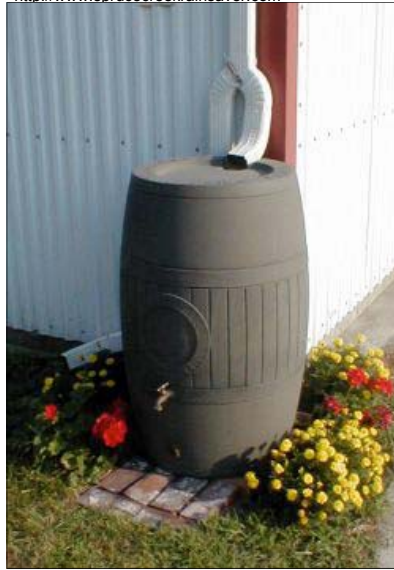
A Rain Barrel connected to a Downspout
