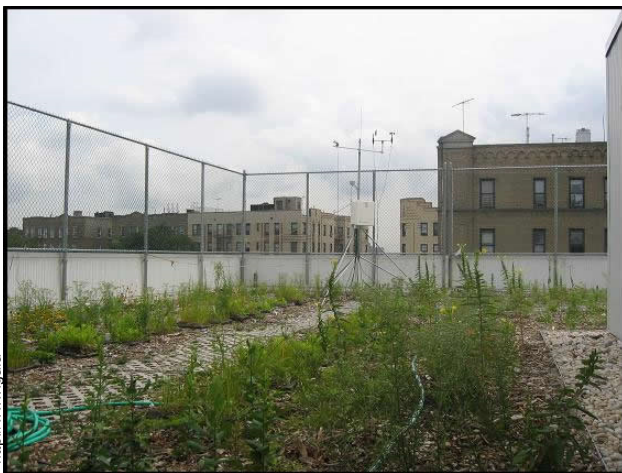
Green Roof at Saint Simon Stock School in the Bronx
